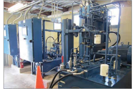
A control system was required for the setting and monitoring of water levels and new locks for the famous San Antonio River Walk excursion boat tourist attraction. This involved design, construction and start-up of three power units and two remote operator panels for controlling the lock system.
