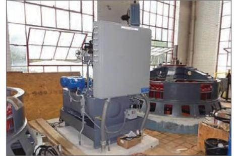
*Sorensen Systems designed and built turbine control panels and balance of plant control panels as part of the Spartanburg Water Treatment improvement project.*
