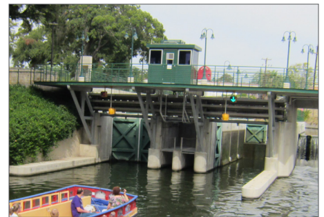
Sorensen Systems and Steel Fab worked together to design, build and install two sets of miter gates and a crest gate at the San Antonio River Walk.
